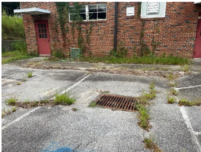
Photograph 21 – Subject Property – Typical Storm water Drop Inlet
